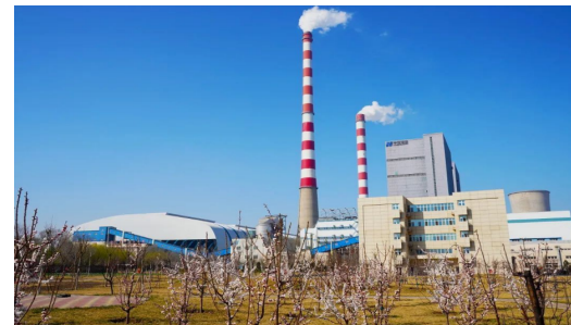
Tianjin Yangliuqing Thermal Power Station
