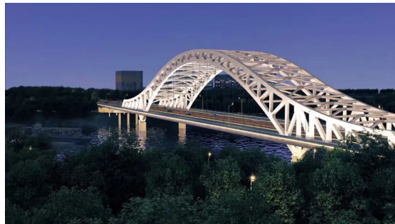
Cross Tuhai River Bridge
