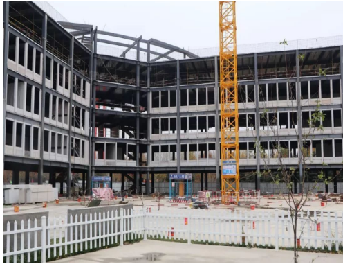
The first provincial prefabricated steel structure school building demonstration project in Linyi City
