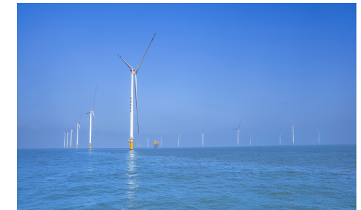
Zhanjiang Wind Power Plant
